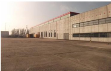
fig. 12_ Belcrum Haven_ Manitowoc Company
