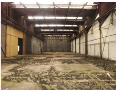
fig. 102_ Interior of building next to the offices of the Backer and Rueb
