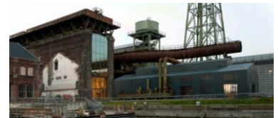
fig. 47_ Pump house on the right, Steam Blower House on the left
