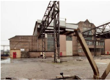
fig. 137_ Structure going out of the building at the road side- 1996
