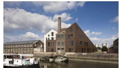
fig. 63_ Barking Watermill, new façade on the river side
