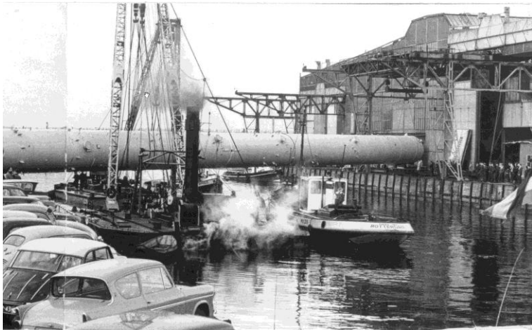
fig. 183_ Heavy transport from the factory Backer and Rueb; 1987
