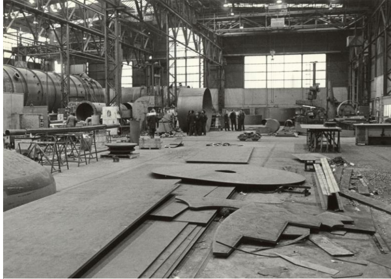
fig. 186_ Interior of the factory in 1983 - Looking to the canal side
