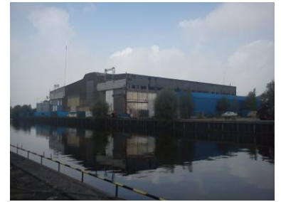
fig. 141_ Façade with a variety of materials
