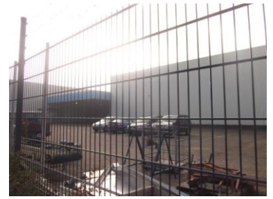
fig. 103_ Private area of contemporary industrial building
